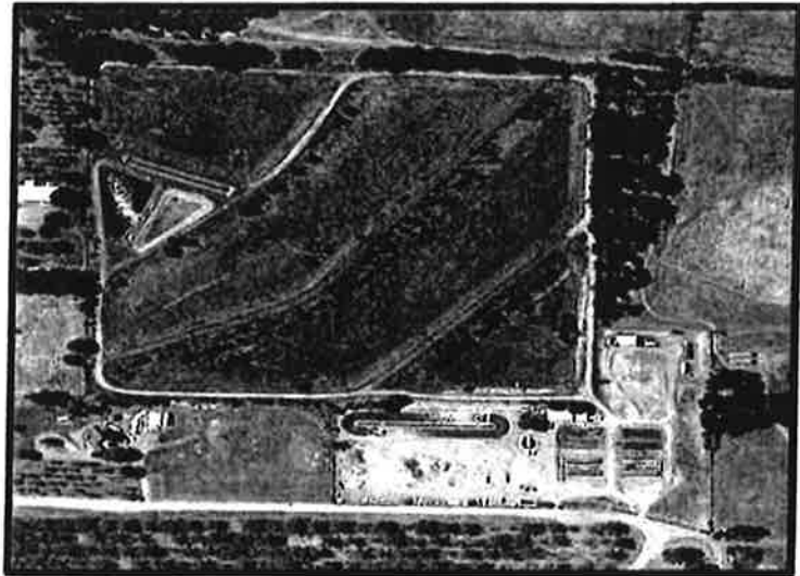
Figure 3, Wastewater Treatment Plant Aerial
