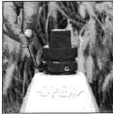
2.) Place the pentagon adapter on and secure with SS set screws. Allen wrench is provided. This leaves you with a standard pentagon to open and close the hydrant as you normally would.
