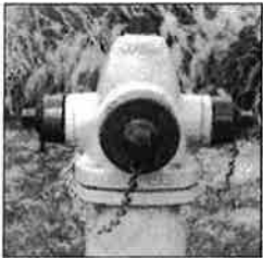
1.) Standard hydrant with a 1-1/2" pentagon (AWWA standard)—unprotected from water thieves!
