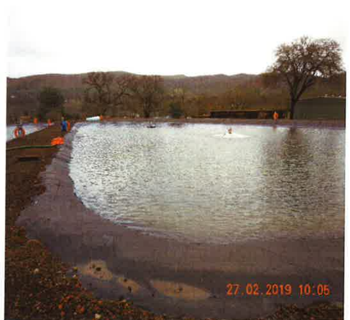
Photo No. 16: Looking east at wastewater aeration pond no. 2.
