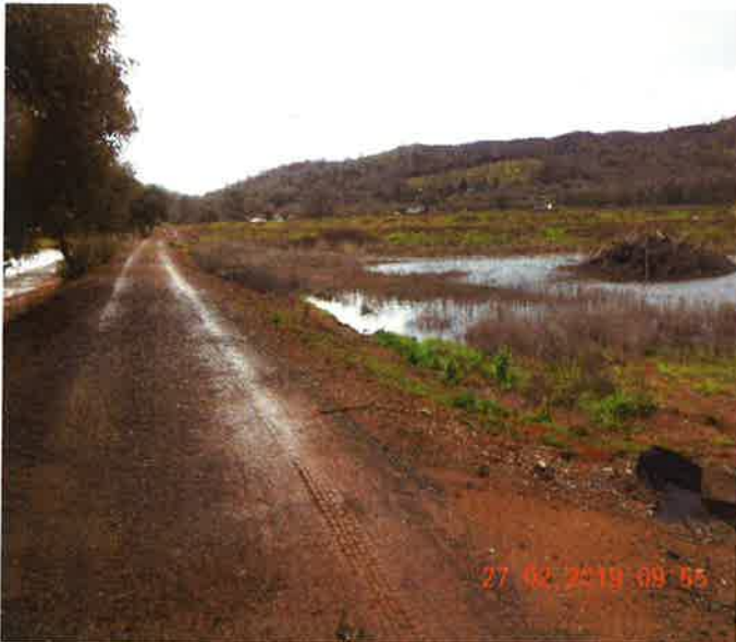
Photo No. 17: Rainwater in one of the four emergency wastewater storage ponds.
