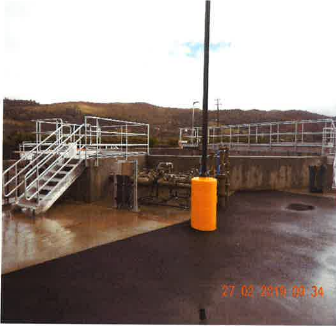
Photo No. 5: Looking east at the newly constructed clarifier.
