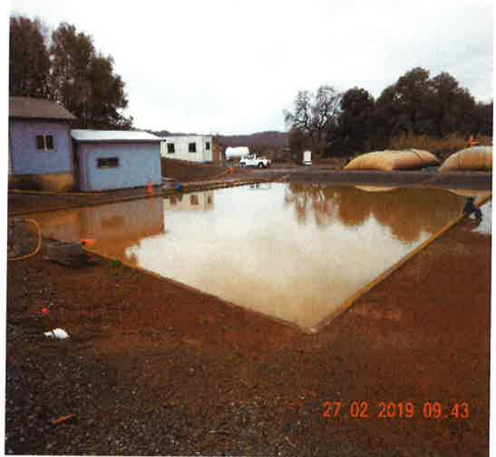
Photo No. 10: Rainwater in one of the sludge drying beds. The water was to be pumped in the treatment plant.
