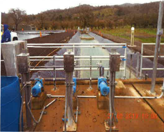
Photo No. 13: Looking south at the chlorine contact ditch.
